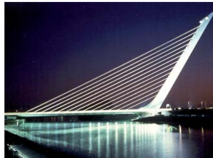
Ryc. 33. Santiago Calatrava, most podwieszony Alamillo w Sewilli, 1990–1992, l_{\max} = 200,0 m [6]
