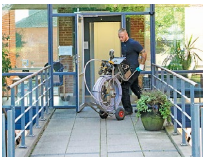
Ryc. 1. Transport systemu Bluelight LED do budynków Rosengaarden Care Home
