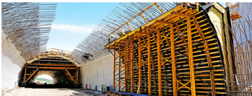
Tunel TS-32, droga S3
