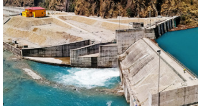
Elektrownia Upper Tamakoshi, fot. Upper Tamakoshi Hydropower Limited
